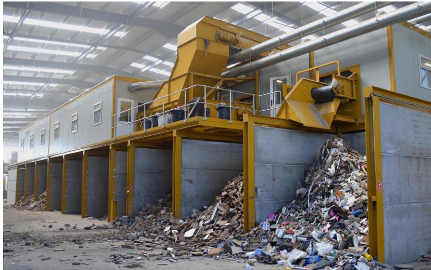
Figure 1: Construction & demolition waste recycling facility
